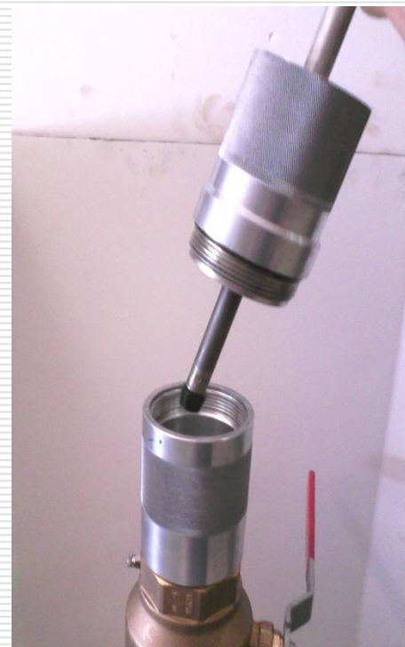
Insert self-tapping plug
